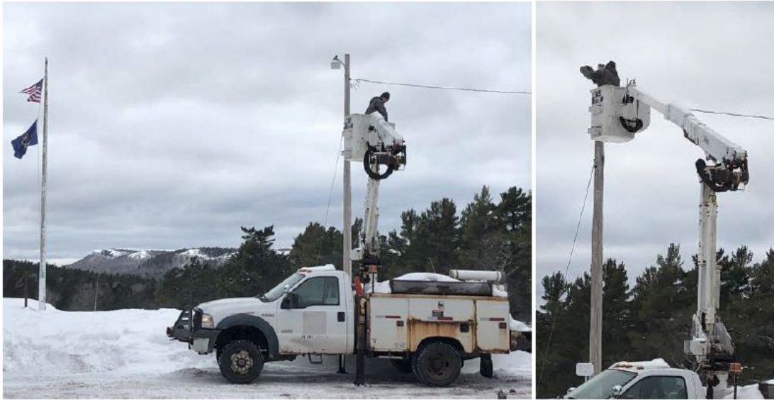
Hole 1 / Brockway Webcam, with the Hole 1 street light and cabin road street lights replaced with Dark-Sky Compliant light fixture (note: even with more street lights working on the cabin road, there is less light pollution on the golf course)
