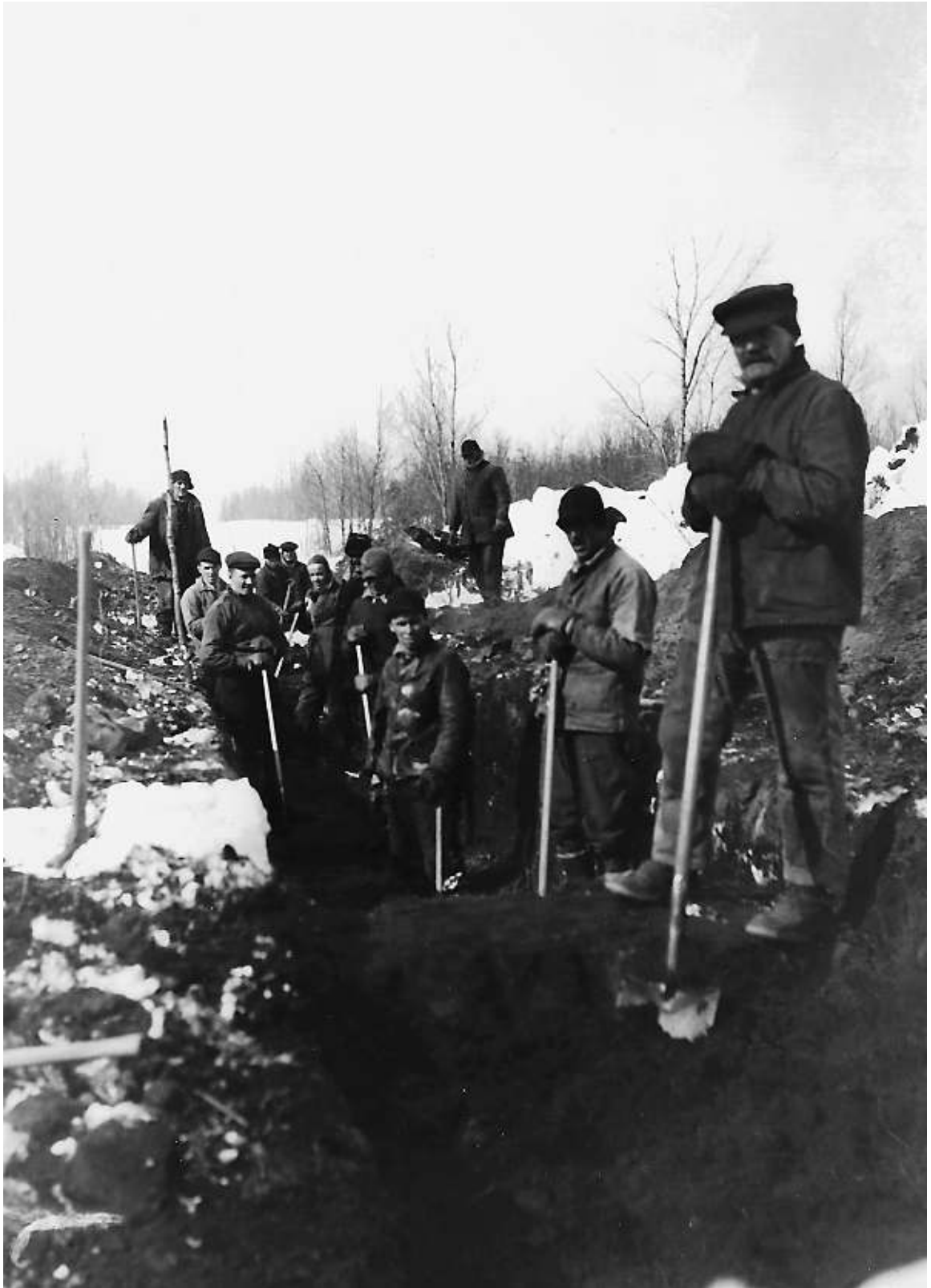
Workers digging a trench during the construction of the Clubhouse - date unknown (Source: Paul La Vanway / Michigan Tech Archives)
