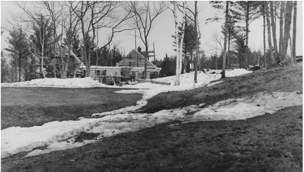
Construction of the second group of WPA funded Cottages in 1936 (Source: Paul La Vanway / Michigan Tech Archives)
