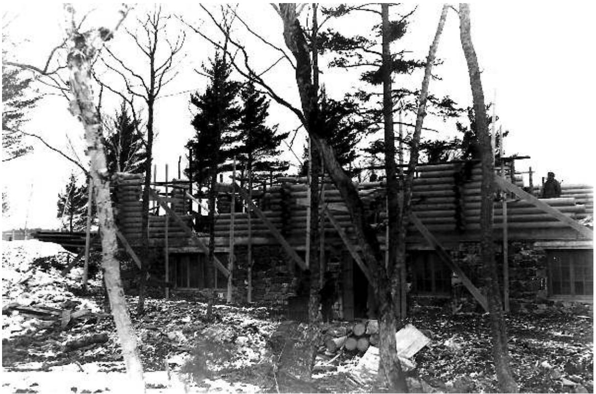
Construction of the Clubhouse building - 1934 (Source: Paul La Vanway / Michigan Tech Archives)
