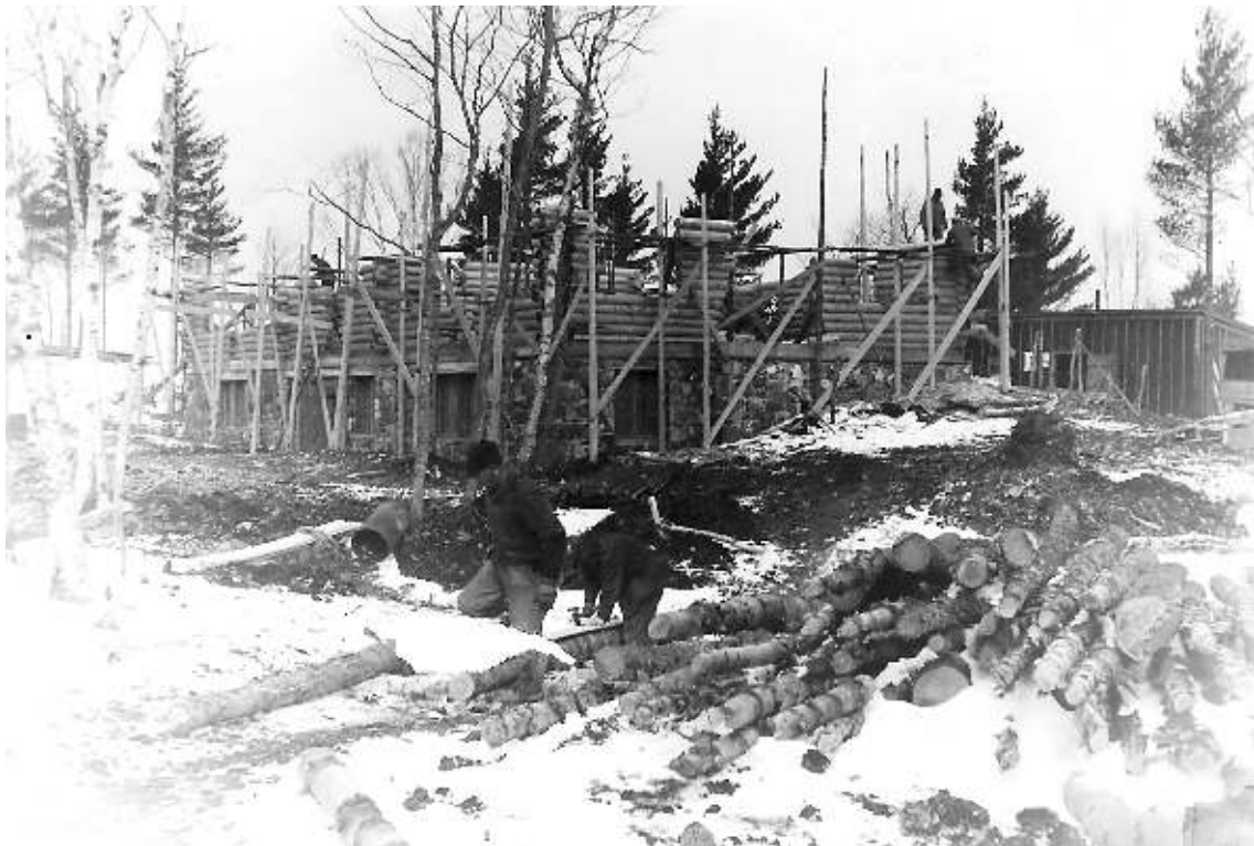
Construction of the Clubhouse building - 1934 (Source: Paul La Vanway / Michigan Tech Archives)
