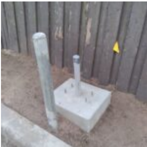
June 8th, 2022 – Platform and bollard installed (photo 2).
