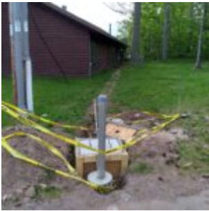
June 9th, 2022 – Platform and bollard installed (photo 2).
