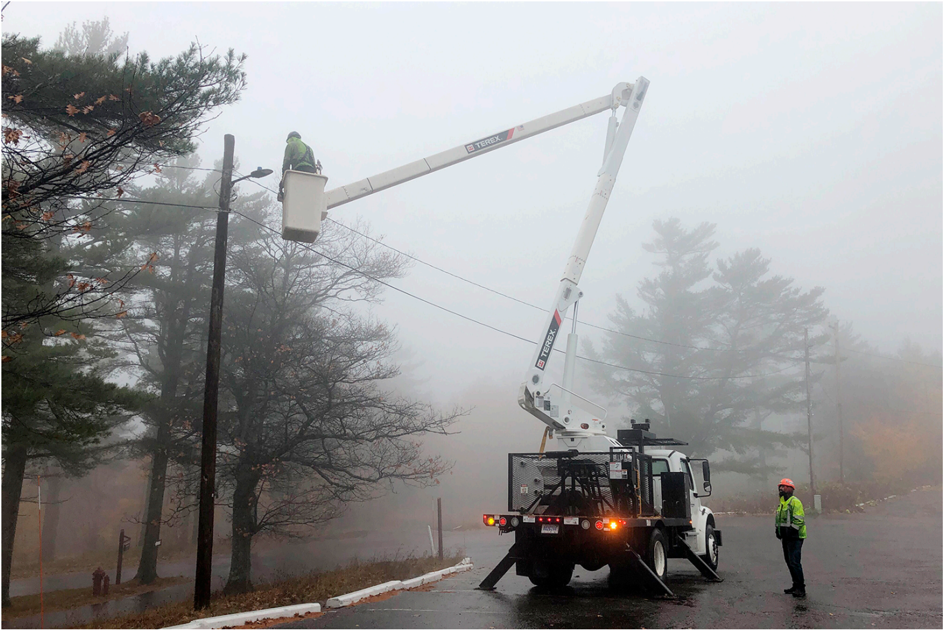
A boom truck installing the Wifi modules on the street lights
