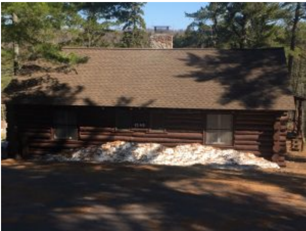
Cabin 25 – New roof
