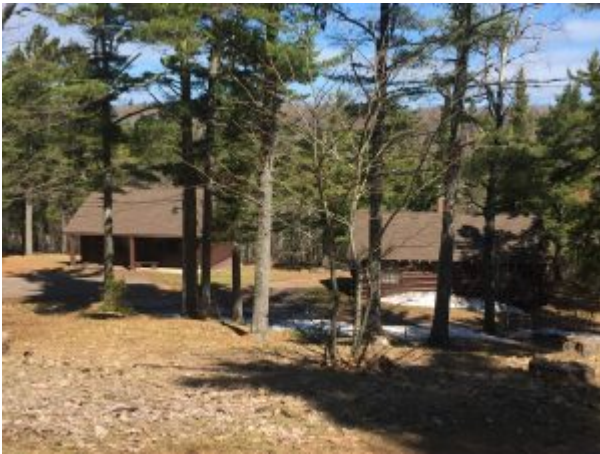
Cabins 22/23 – New roofs
