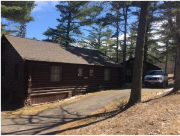
Cabin 24 – New roof
