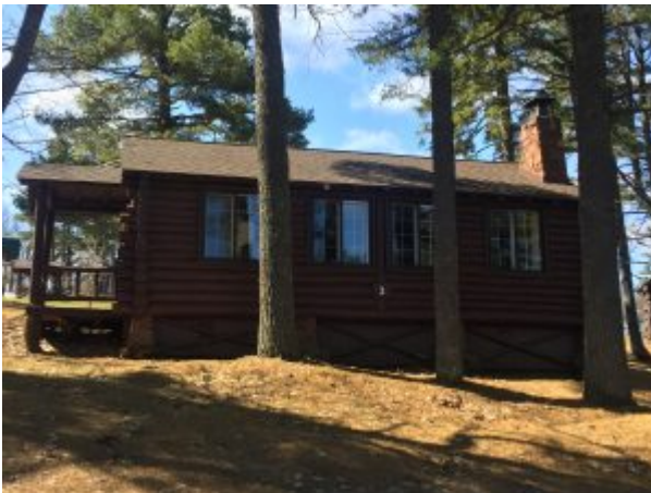
Cabin 3 – New roof in 2019
