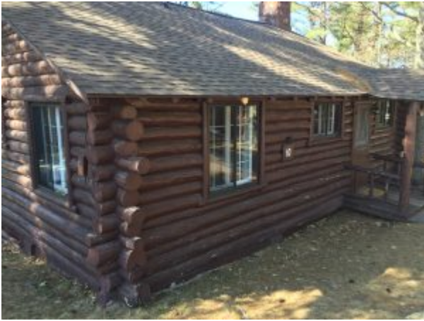
Cabin 10 – New roof in 2019
